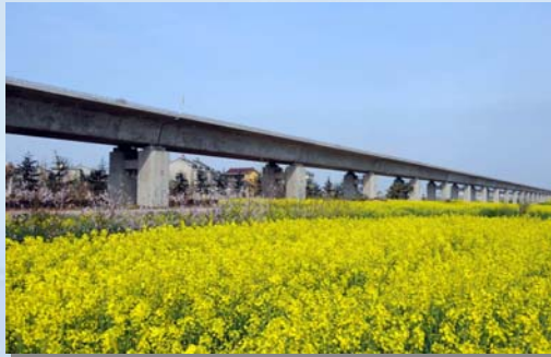
Beijing-Shanghai High Speed Railway
